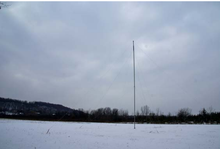
Vertical Antenna (with 48 radials) This is the Antenna David will use with "GWEN"
